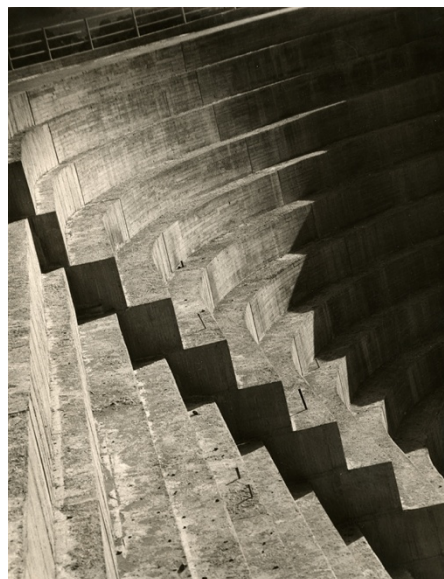
Alma Lavenson, "Calaveras Dam" 1932.
